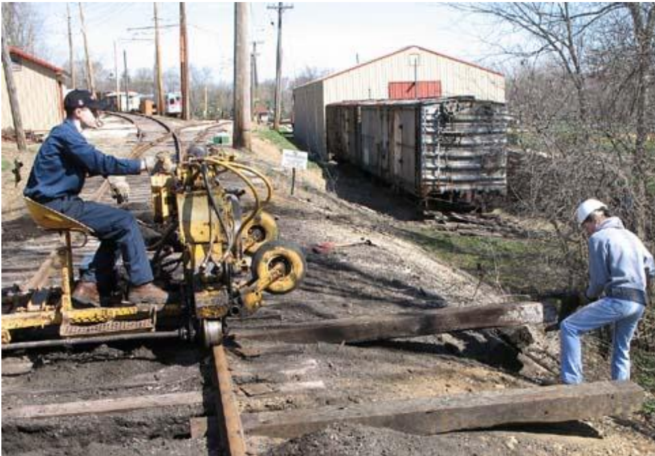
Matt DelGuidice operating the tie inserter as Chris Nelson guides in the tie with the inserter hook.
