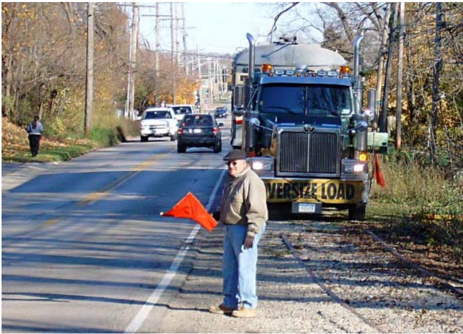
Member Stan Nettis flagging traffic by on Illinois Route 31 ensuring a safe operation. Don MacBean
