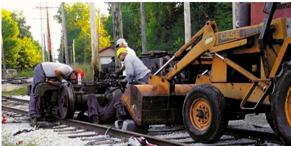
From left to right, Fred Lonnes, Chuck Galitz, Joe Hazinski and Joe Solinski installing the refurbished "#1" motor. Don MacBean
