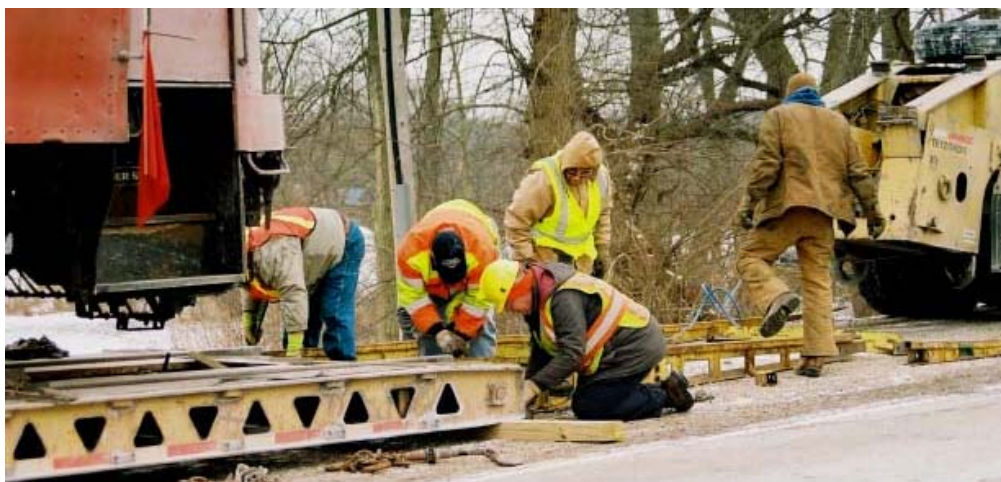
Fred Lonnes, Silk Road escort Driver, Chuck Galitz, Joe Hazinski and Silk Road driver, Jay Jackson readying the ramp over which CA&E 458 will finally reach its new home rails.
