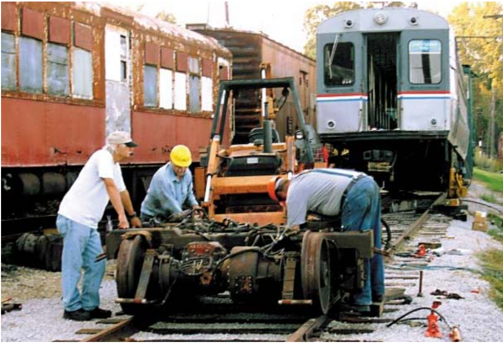
Joe Solinski, Joe Hazinski and Fred Lonnes work on the installation of the refurbished motor. Don MacBean
