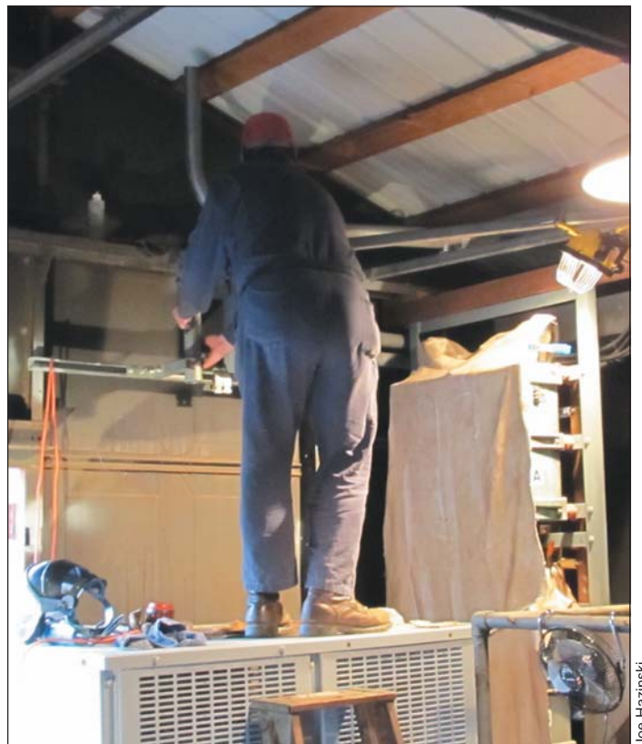
Below: Once the transformer was in place Chuck Galitz started installing the conduit for the wiring so that the sub station can go back on line. Through everyone's efforts traction power was available for inspection work, crew qualification and, of course, opening day on May 8 th .
