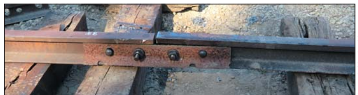
The joint bars have been applied and now gauging and spiking will begin.
