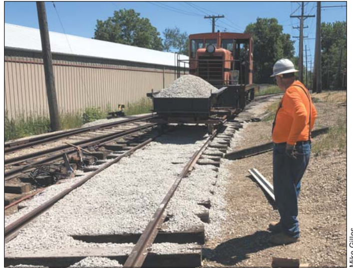
The next weekend Fred Lonnes watches as Locomotive 5 pushes the EZDumper down Track 0 to begin the ballasting process.
