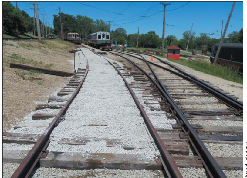
The ballast has now all been delivered to Track 0 so that the first tamping can be done.
