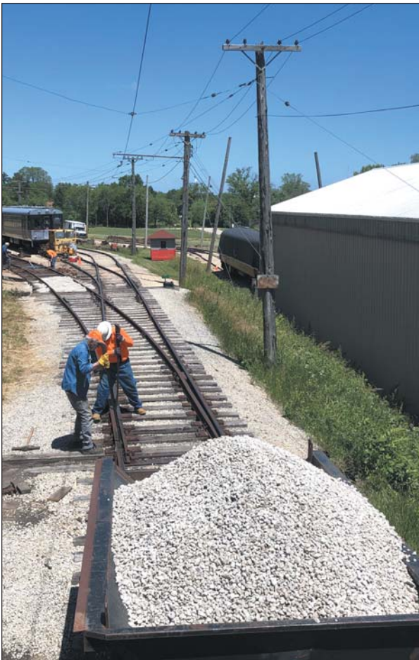
Fred and Mike bar over Switch 21 as the switch stand was yet to be connected, so 5 can deliver another load of ballast.
