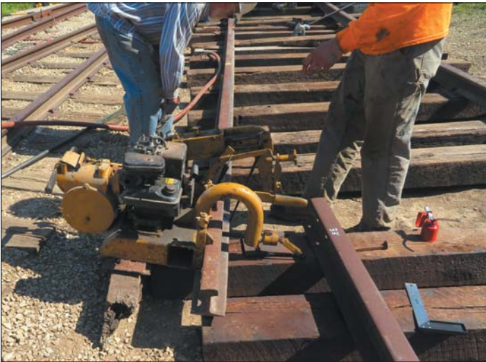
Our Briggs & Stratton powered Racine rail saw is cutting the excess off of one of the two rails that needed to be trimmed.
