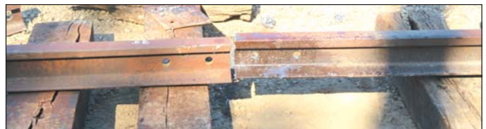
The ends of the freshly cut rail have been ground smooth and now await joint bars.
