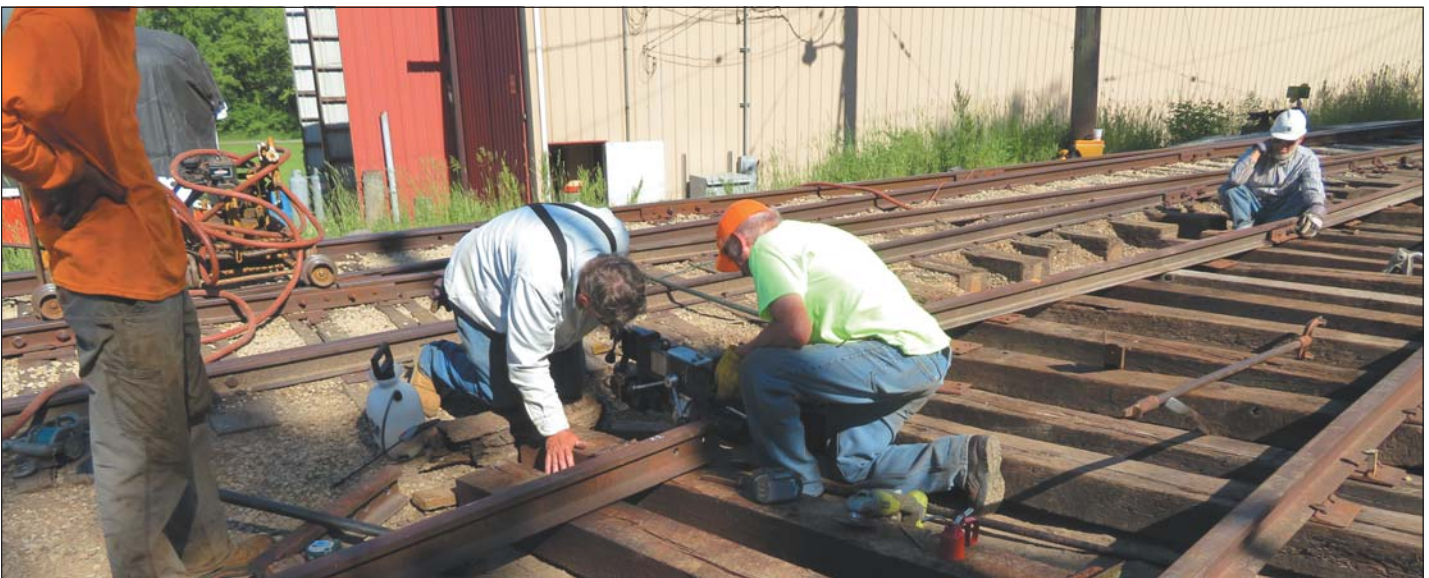
Chris watches as Fred and Mike Gilles set up Fred's electric rail drill which will bore out the holes for the joint bars.
