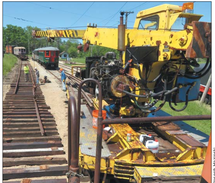
CTA S-314 is putting down one of the rails recovered from the museum's supply on May 31 st .
