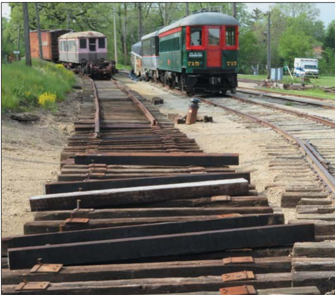
The ties and tie plates are in the process of being laid out while CNS&M 715 and CTA 43 are laid up ahead of MUNI 1030 on Track 1.
